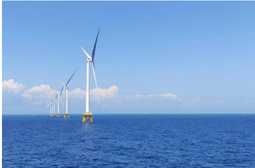
Installation works of the offshore wind farm in Huizhou, Guangdong
