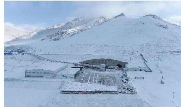
Tianshan Shengli Tunnel of the Urumchi-Yuli Expressway
