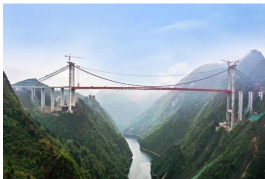
Guiyang - Huangping Expressway Baoshan Super Bridge
